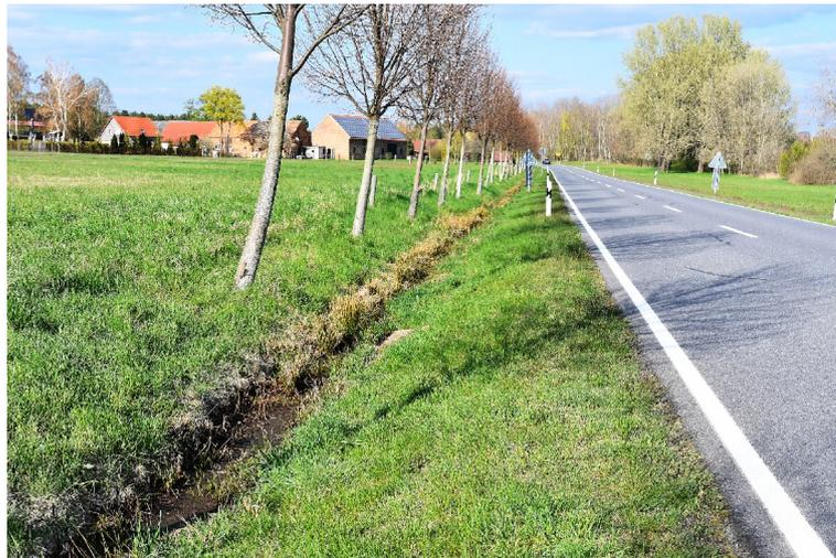
Figure 21: Existing roadside ditches could be converted into infiltration swales.
